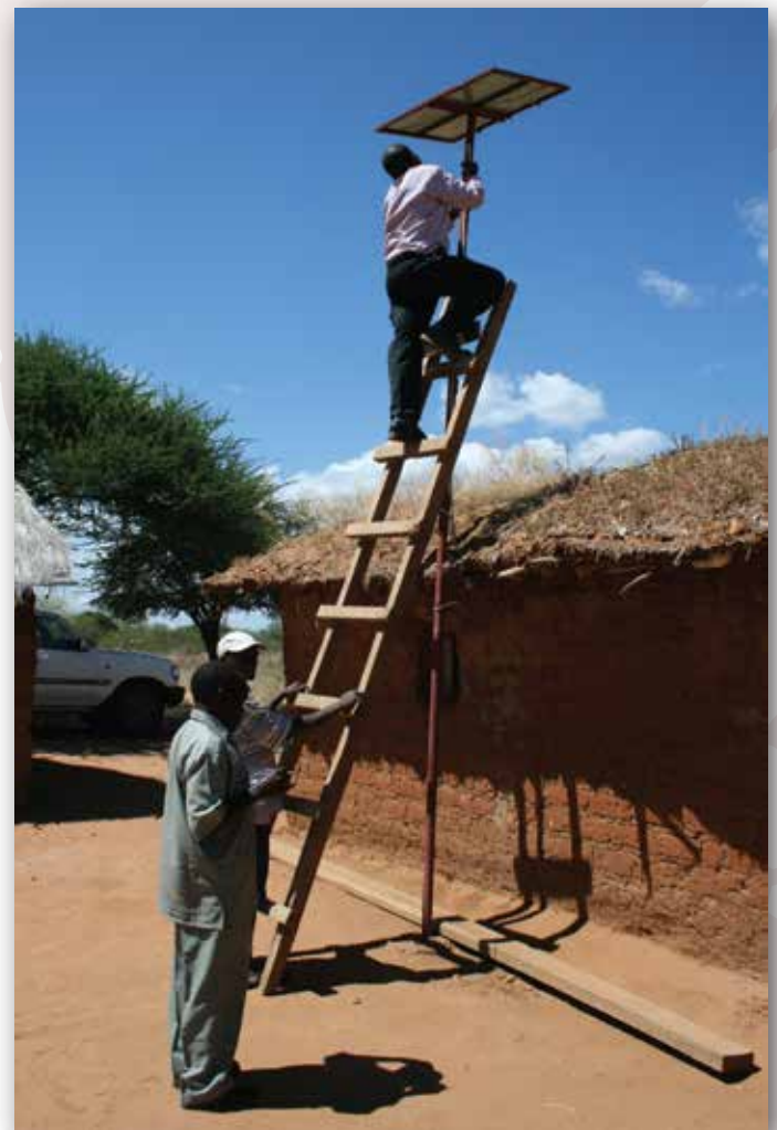
Installing a small solar PV panel
